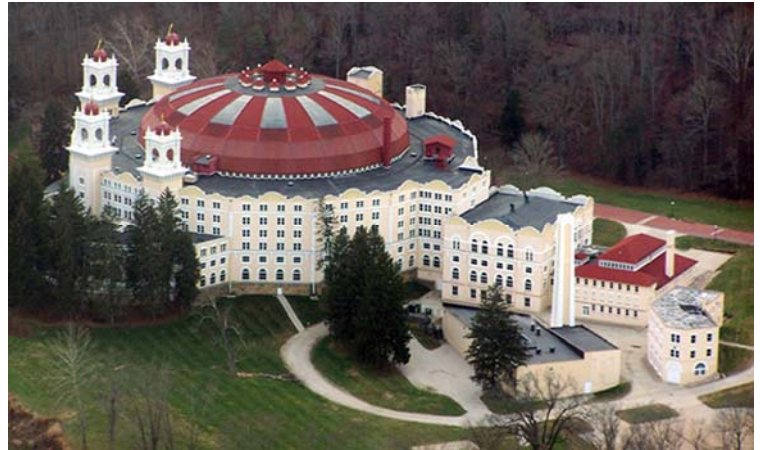
An aerial shot of the newly-restored West Baden Springs hotel
